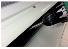
TAKING CARE NOT TO OVER TIGHTEN - Bend the rail to the contours of the van (the Combi-Rail is made from a malleable alloy to make this process easier) When the front half is secured do the same from the middle of the rail towards the rear of the van TAKING CARE NOT TO OVER TIGHTEN.
